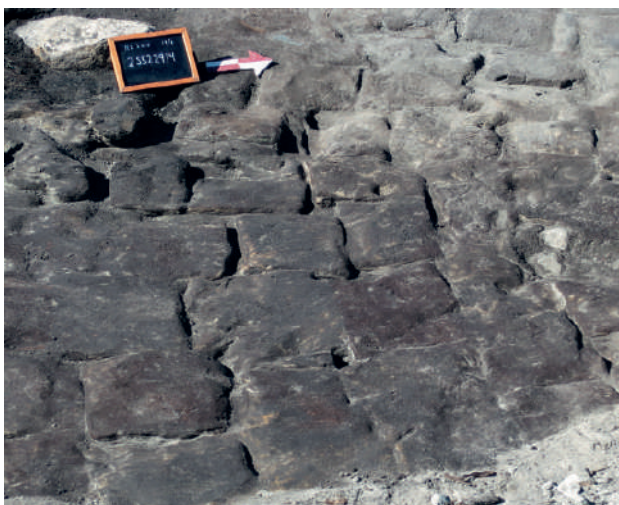
Figure 4. Example of a one-layer turf construction underneath a floor constructed 1470–1480 in Nya Lödöse, Sweden (Photo Jonathan Pye, cf. Morner et al. 2021: 95).
