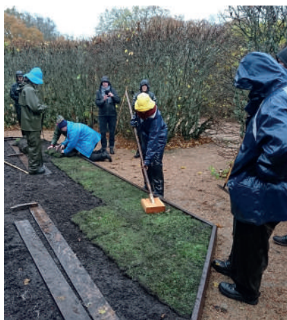
Figure 3. Experimental laying of pasture turf and use of a turf beater in the Mollet lawn, Gunnebo 2017 (Photo Joakim Seiler, cf. Seiler 2020: 98).
