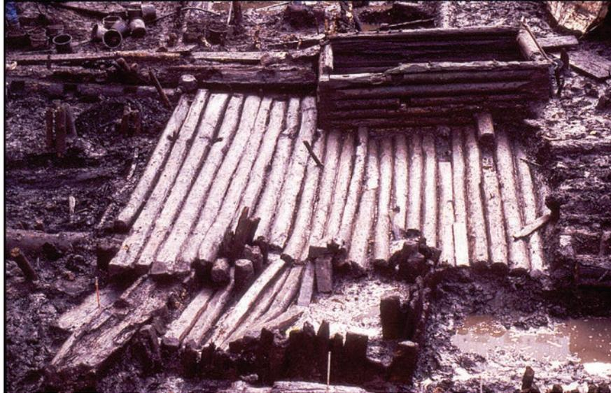
Figure 6. In Mätäjärvi quarter, a yard between two buildings was carefully paved with logs in the 1400s. The pavement covered an area of 43 m<sup>2</sup> (Seppänen 2012b, p. 359–365, original photo: The Museum Centre of Turku.).
