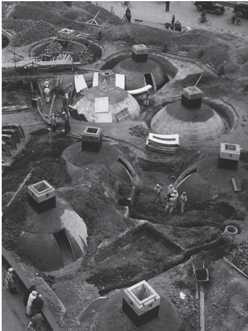
Figure 9. Photo from 1944 showing the construction work of air raid shelters somewhere at Rådhuspladsen. They explain the fragmentary patterns seen in area 2. Photo: Unknown. Copenhagen City Archive.
