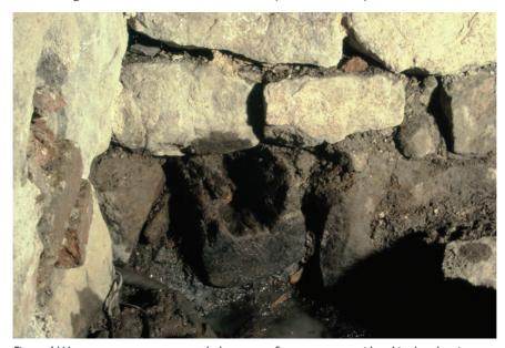
Figure 4. Wastewater management and placement of sewers was considered in the planning and construction of buildings, too. A masonry building from the 15th century was provided with a timber sewer leading the waters to the gutter of the adjacent street (Seppänen 2012b, p. 882, original photo:The Aboa Vetus & Ars Nova Museum, Turku).
